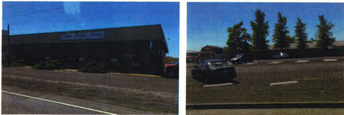
Figure 6: Examples of Existing Landscape Conditions
