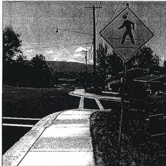
Recently constructed sidewalks and crosswalks on Cherry Street.
