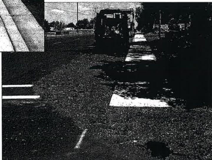
Many sidewalks end abruptly (above) or need a short pavement connection to crosswalks (right).
