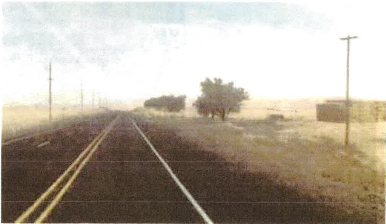
Potential turn around location
