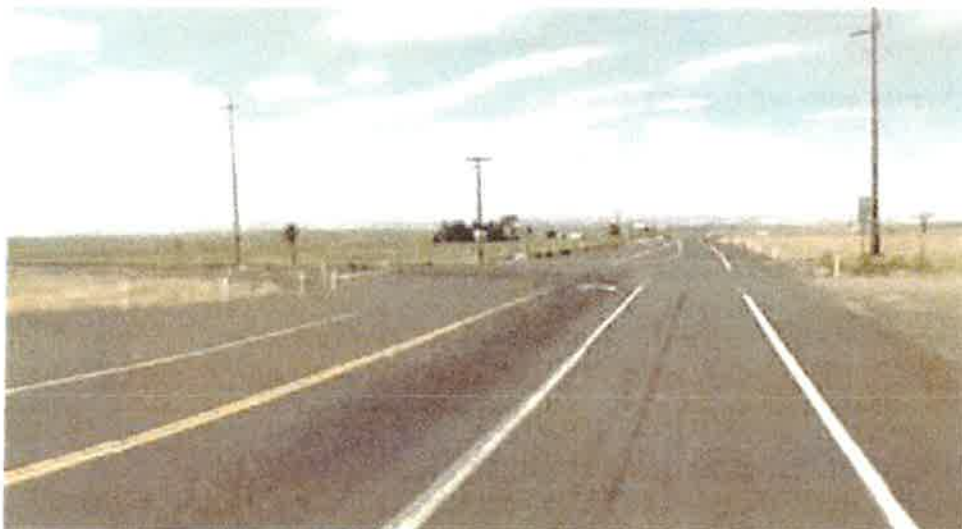
Looking south west on Hwy 11. Loads will come from 331 from the road entering on the left.
